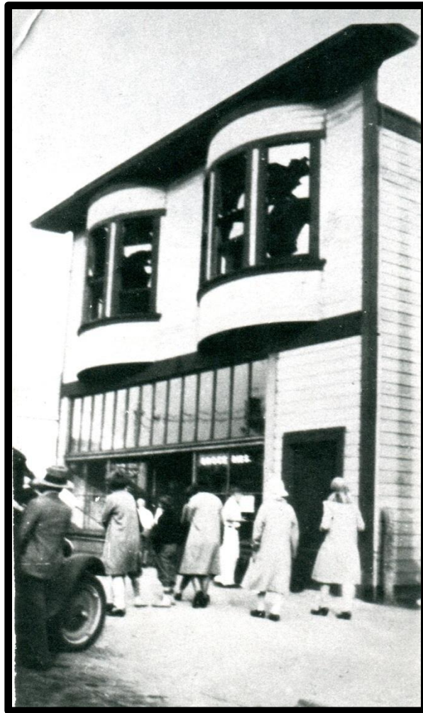
1261 B Street is where the shootout took place. Notice the broken windows on the second floor. The building was torn down in the 1960s.
