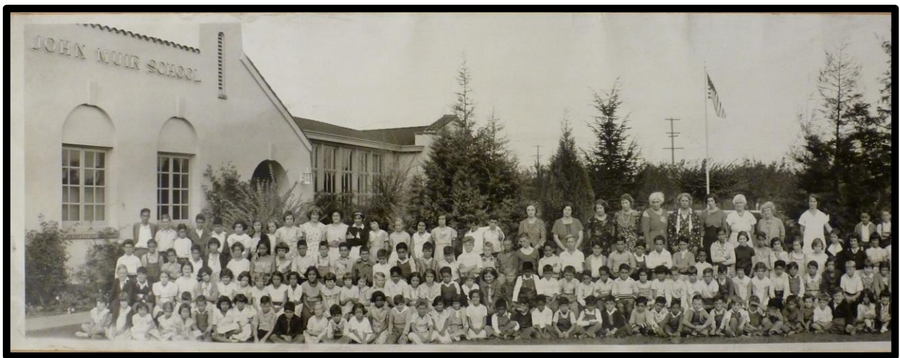
John Muir School as it appeared in 1934, just about a year before it was destroyed by fire.
