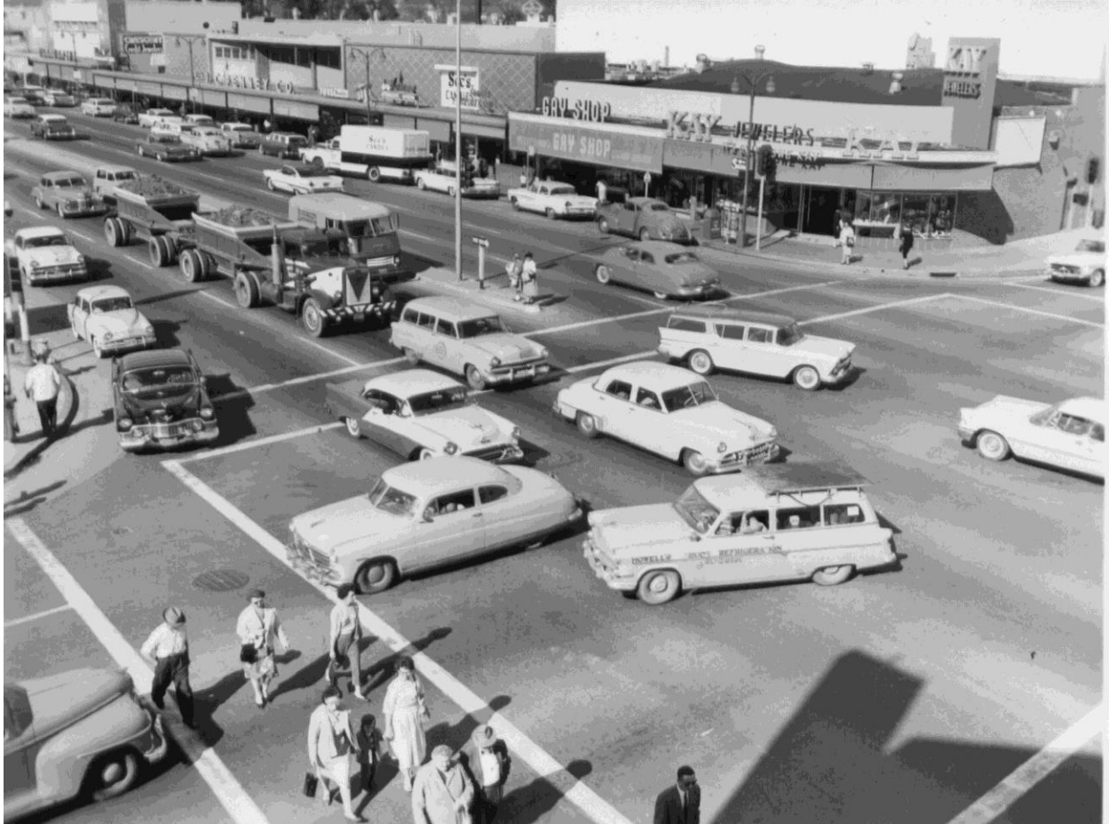
The rebuilt Foothill Boulevard store in the upper left, February 26, 1960.
