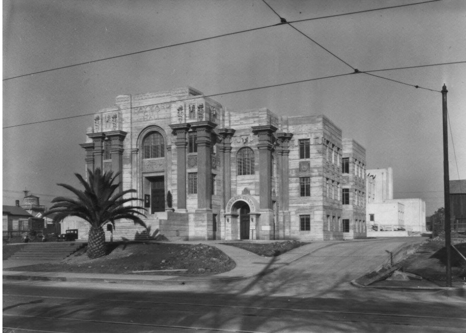
City Hall under construction, summer 1930.
