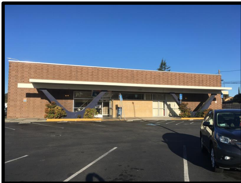
The Castro Valley Post Office as it appears today.
