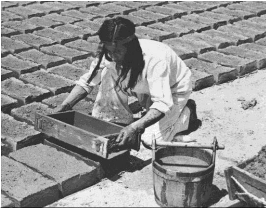
Adobe bricks were made by hand. They were used to build the mission and other buildings. It was hard work to mix the dirt, water, and straw to make adobe.
